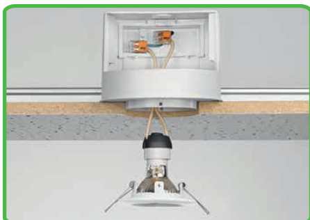
Individual design of low-voltage lighting systems.
