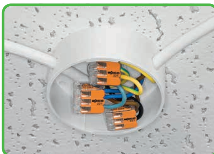
Lighting distribution in ceiling canopy
