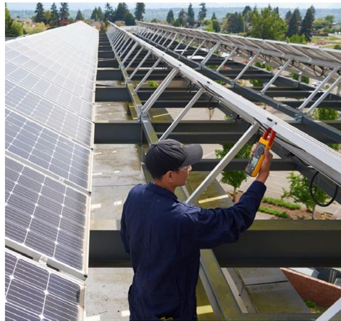
Troubleshooting is a vital part of the professional solar technician's skill set. Here the technician takes readings at the rear of a PV panel with a Fluke 393 FC.
