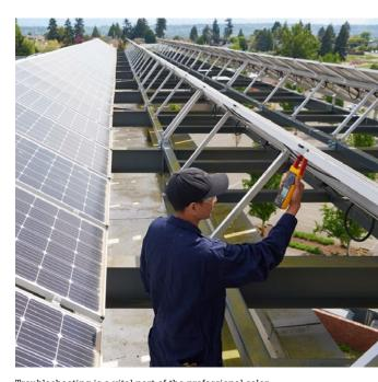
Troubleshooting is a vital part of the professional solar technician's skill set. Here the technician takes readings at the rear of a PV panel with a Fluke 393 FC.
